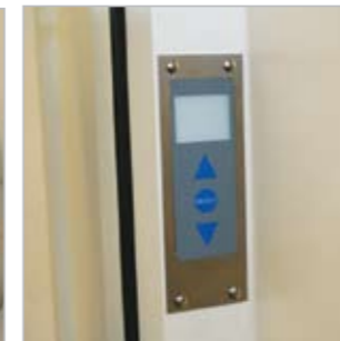
Flush-mounted switch
