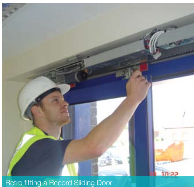
All in one control unit with monitored battery backup
